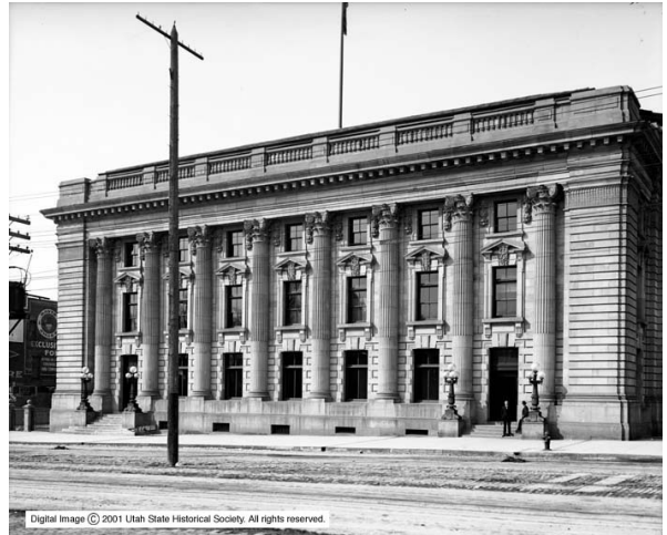
Post Office and Courthouse Building* 1907
